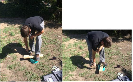
Photos demonstrate installation of beveled collar. We recommend Trex or similar plastic composite decking rather than the wood lumber shown here, and a 3 lb mallet rather than the claw hammer shown here.
